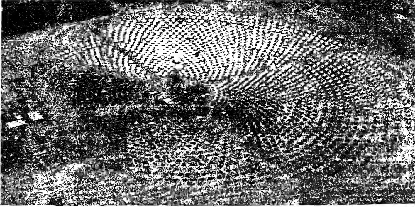
This is Solar One the McDonnell Douglas station in the Mojave desert. More than 1800 heliostats reflect the sun's rays to the central receiver. The heat converts water to superheated steam which drives a turbogenerator able to generate up to 10 megawatts of electricity. The company believes that experience gained with this plant may lead to a wide variety of solar plants in the U.S.
